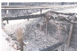
Photo 41: Pigeon Gully Bridge, 12.1.20, Peter Sorensen
