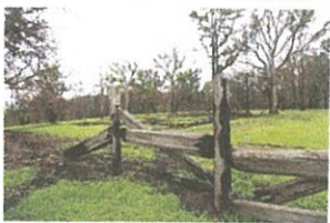
Photo 75: Old Woolla Stock Yard Ruins, 2.2.20, Peter Smith The yards were a showpiece of the hard work and toil by the Davis women who built them in the 1950s out of red gum which they cut, snigged, split and erected with hand tools. Some of the rails were 600mm thick and so heavy that two men would struggle to lift. Black lines on the ground are all that's left.
